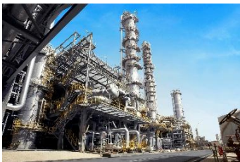
Petroleum and Petrochemicals
